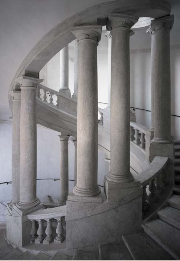
Francesco Borromini, Palazzo Barberini, helical staircase, Rome.
